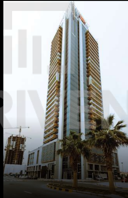
Al Manarah Tower JVT Dubai
