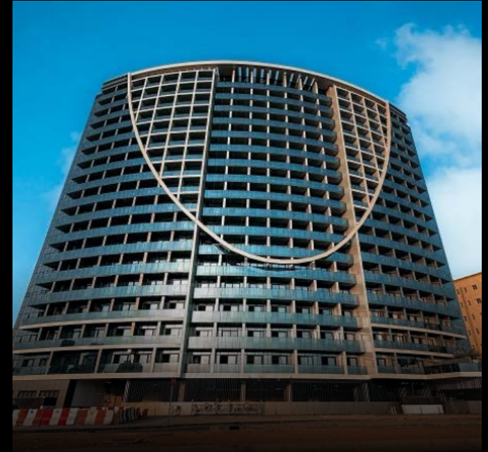
The V Tower Dubai Land
