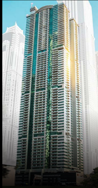
Marina Pinnacle Tower Dubai Marina
