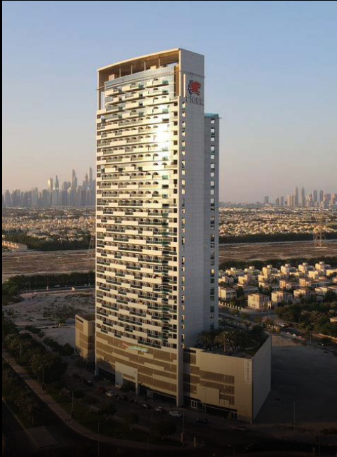
Al Jawahara Tower JVT, Dubai
