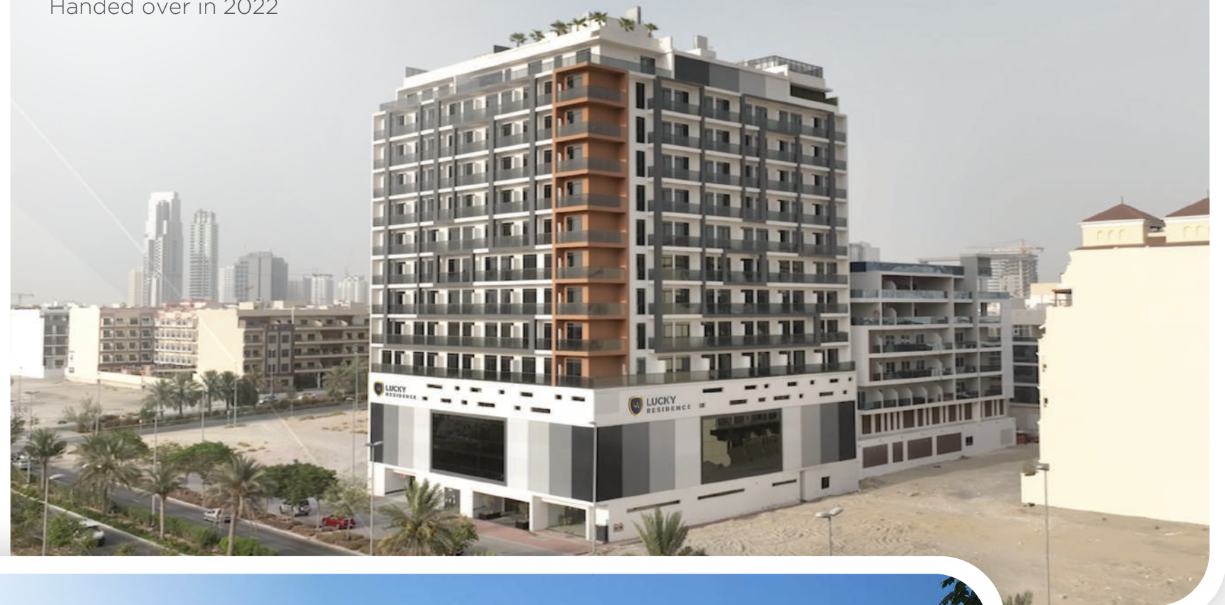
Lucky Residence Handed over in 2022
