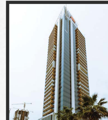
Al Manarah Tower JVT, Dubai
