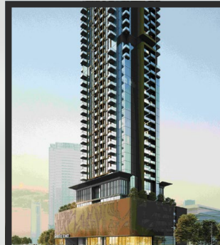
Seslia Tower JVT, Dubai
