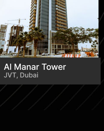
Al Manar Tower JVT, Dubai
