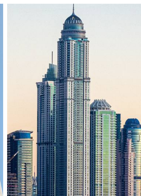
PRINCESS TOWER BY TAMEER HOLDINGS
