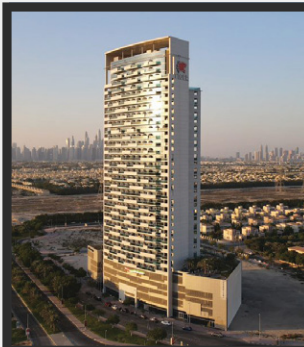
Al Jawahara Tower JVT, Dubai
