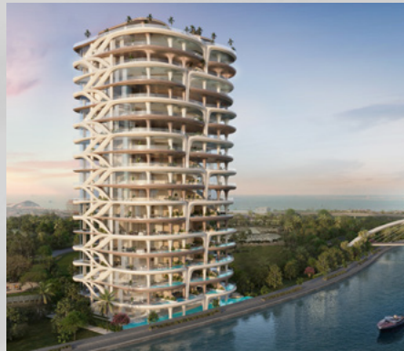
CASA AHS DUBAI WATER CANAL
