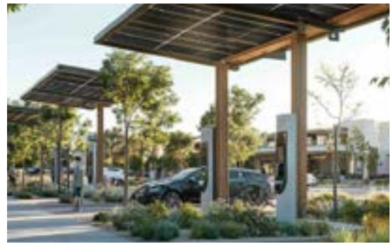
SOLAR CHARGING STATION
